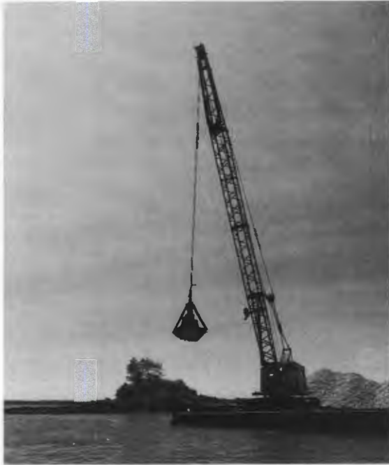
Transporting and deploying surf clam shell at the oyster reef restoration site (2016).
